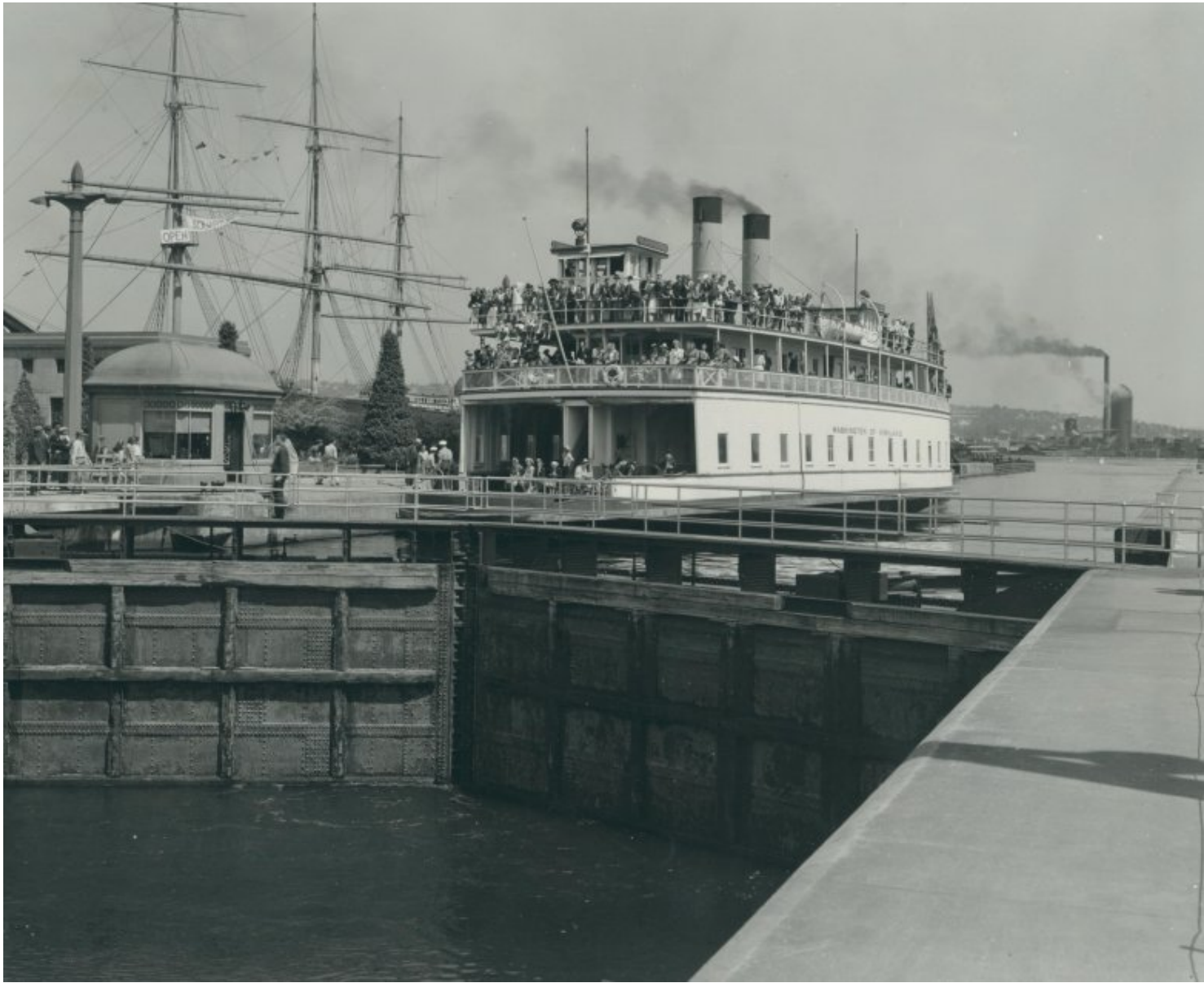
The Washington of Kirkland ferry in the locks.
