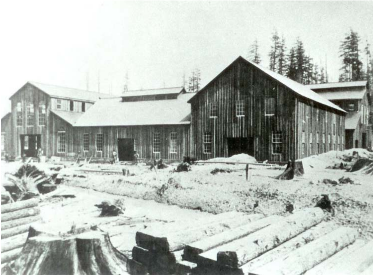
The machine, blacksmith and pattern shops with stacks of railroad ties. The foundry building is behind.
