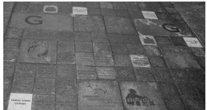
A few pavers had errors and needed to be replaced. Some of the more damaged pavers were also replaced. After a few months of weather and foot traffic they should blend in with the old.
