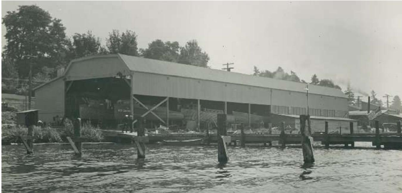
The hulls started at the south end of the building and were built upside down, which was a new technique at that time. When the hulls were completed they were flipped over and the engines were installed, wiring put in, decks put on and the pilot house and deck house installed.
